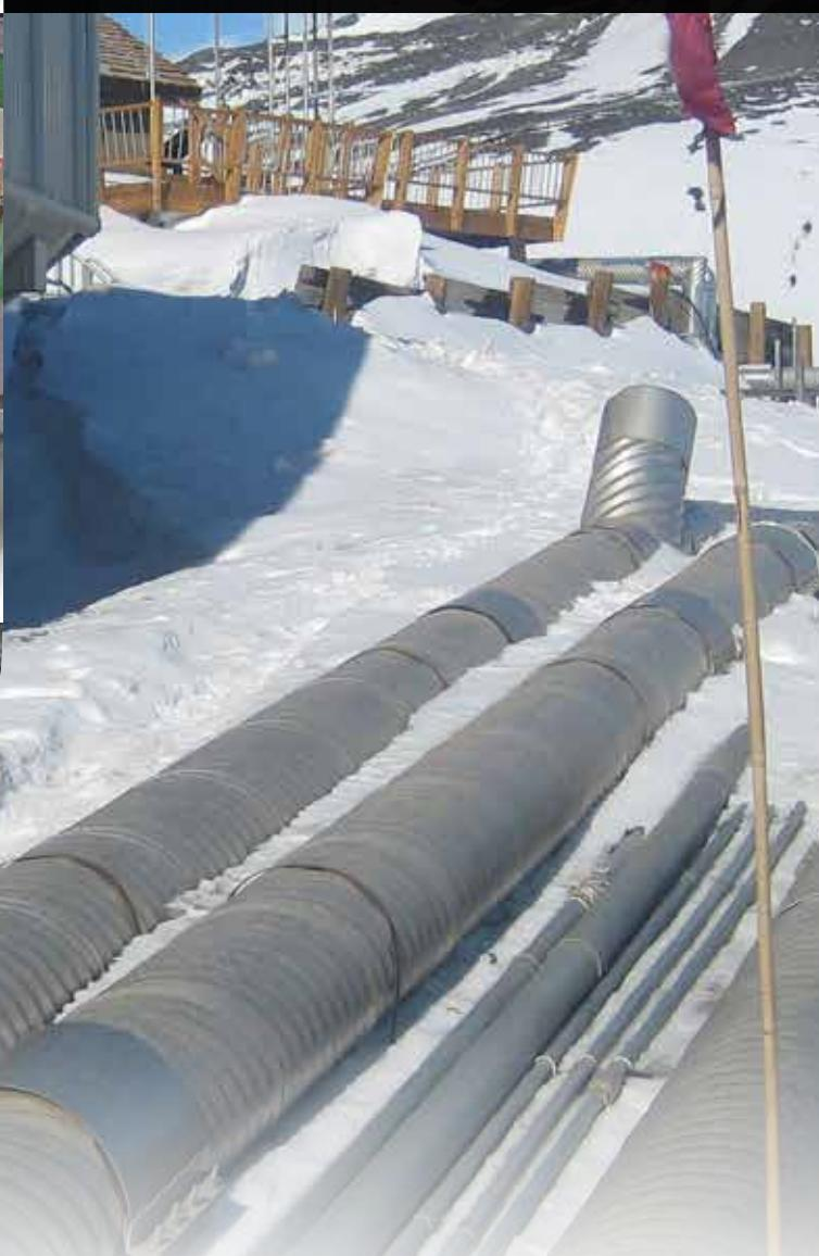
Heat tracing is a system used to maintain or raise the temperature of pipes and vessels in order to avoid fluids from freezing or increase their viscosity.
