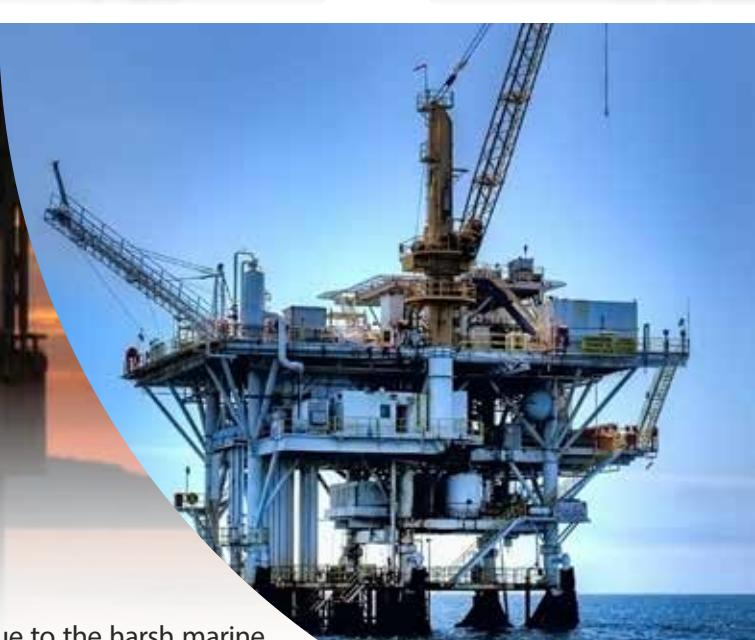
Offshore platforms are constantly exposed to corrosion due to the harsh marine environment. Protection is carried out through aluminium or zinc sacrificial anodes, but when the weight of the structure is critical, an impressed current ICCP system or a hybrid system (impressed current combined with sacrificial anodes) can be the best option.
