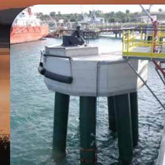
Pontili e infrastrutture portuali / Jetties & harbour facilities
